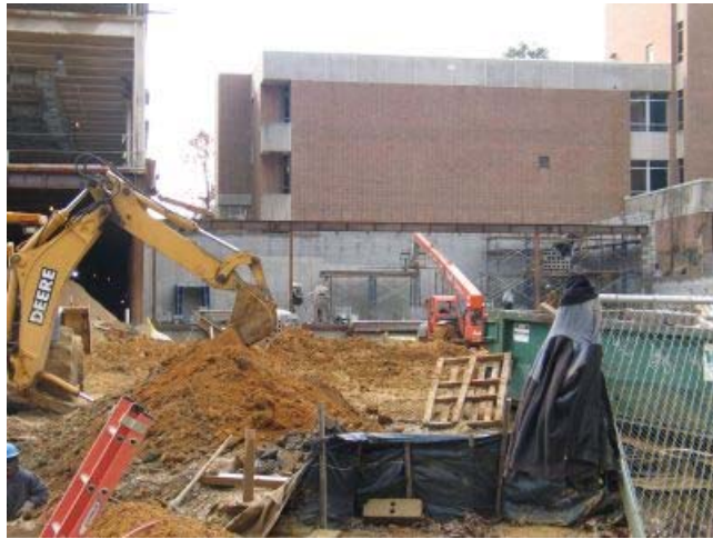
Figure 3.1- Preparation for Excavation
