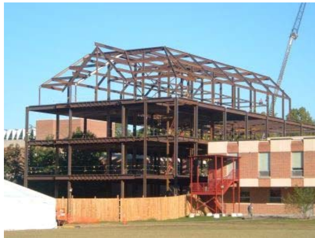
Figure 3.2 - Steel Erection Completion
